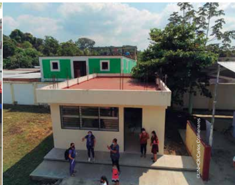
UNHCR supported the remodeling of classroom, restrooms lighting and other facilities at Fernando Montes de Oca school in Tapachula, Chiapas.
